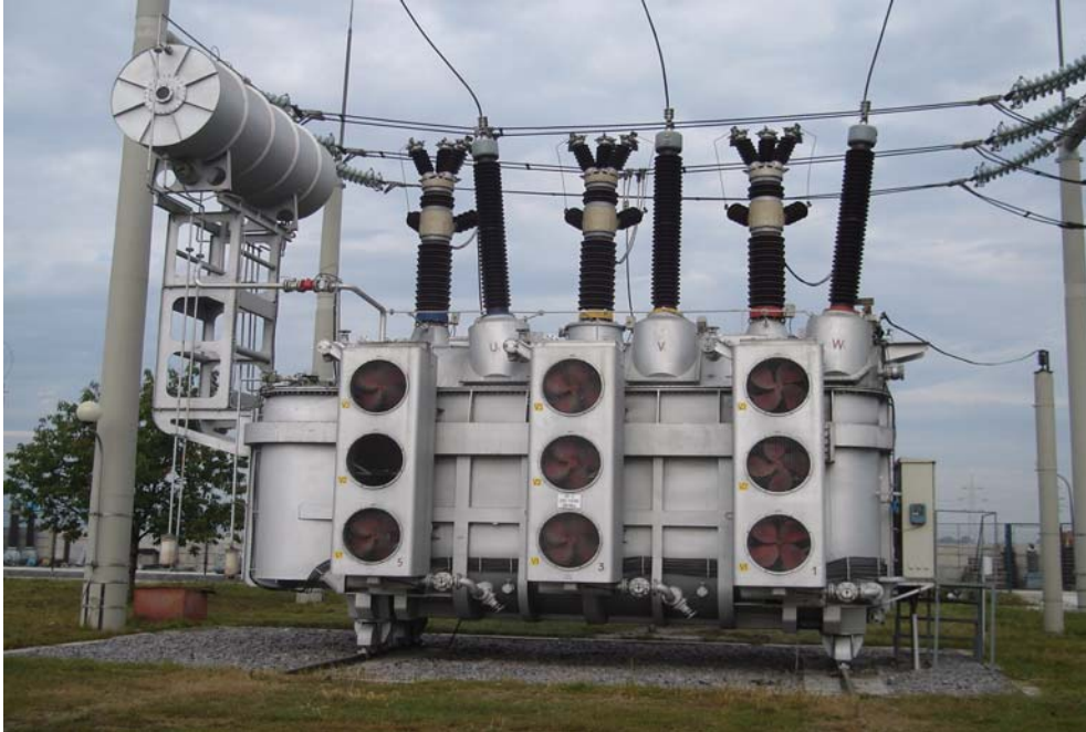
Figure 1. Power autotransformer S=200MVA
