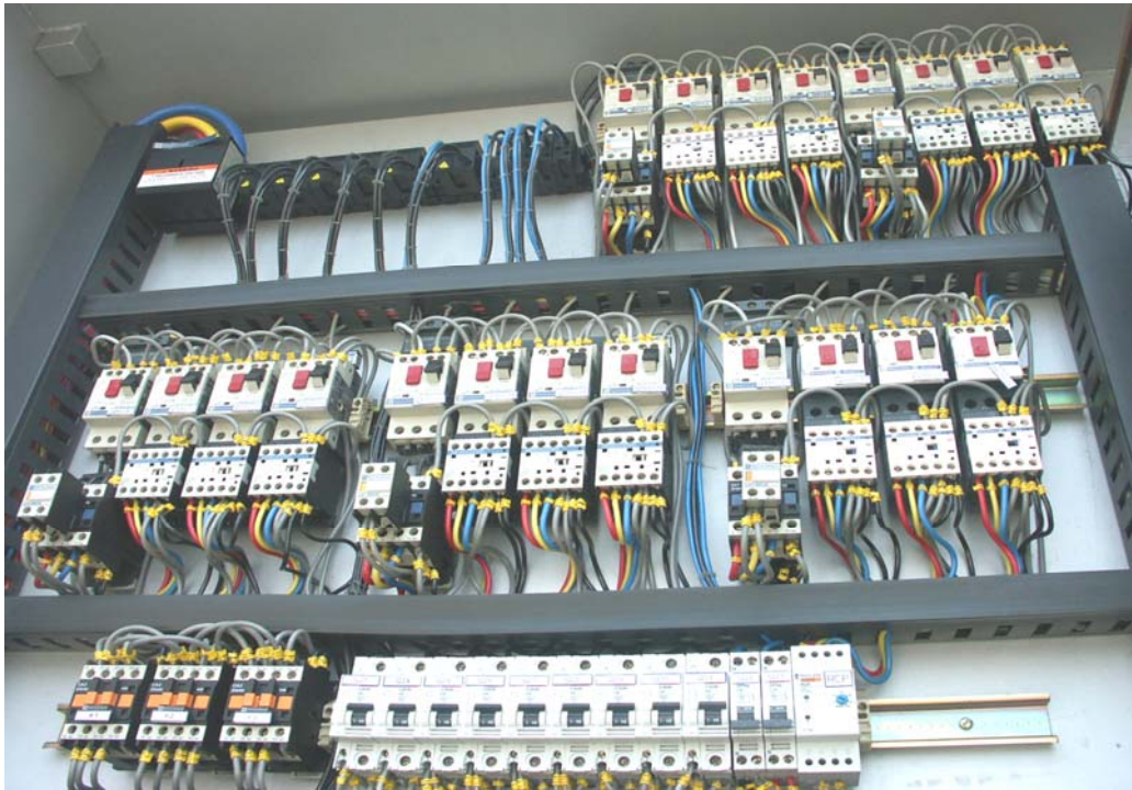
Figure 5. Electric switch box transformer
